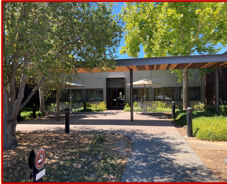
1) CMP front entrance
